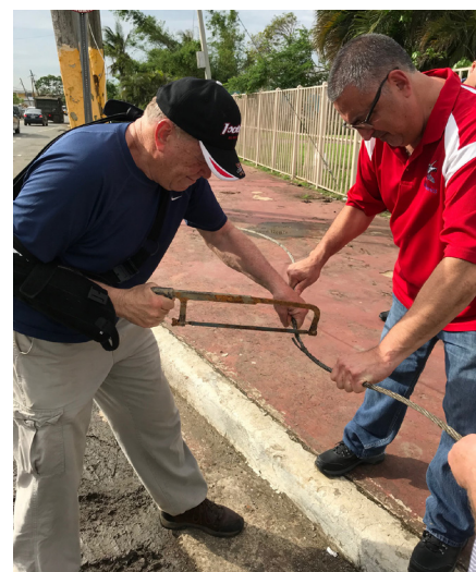
Council team members John Dufay and Mark Zaher cut an electrical ground cable to enable students access to Jose Robles Otero School in Puerto Rico.
