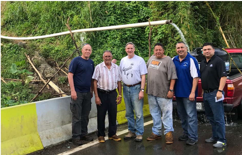
Council team in Puerto Rico working on water supply problems at Cruz-Garcia and Jose-Padin schools.
