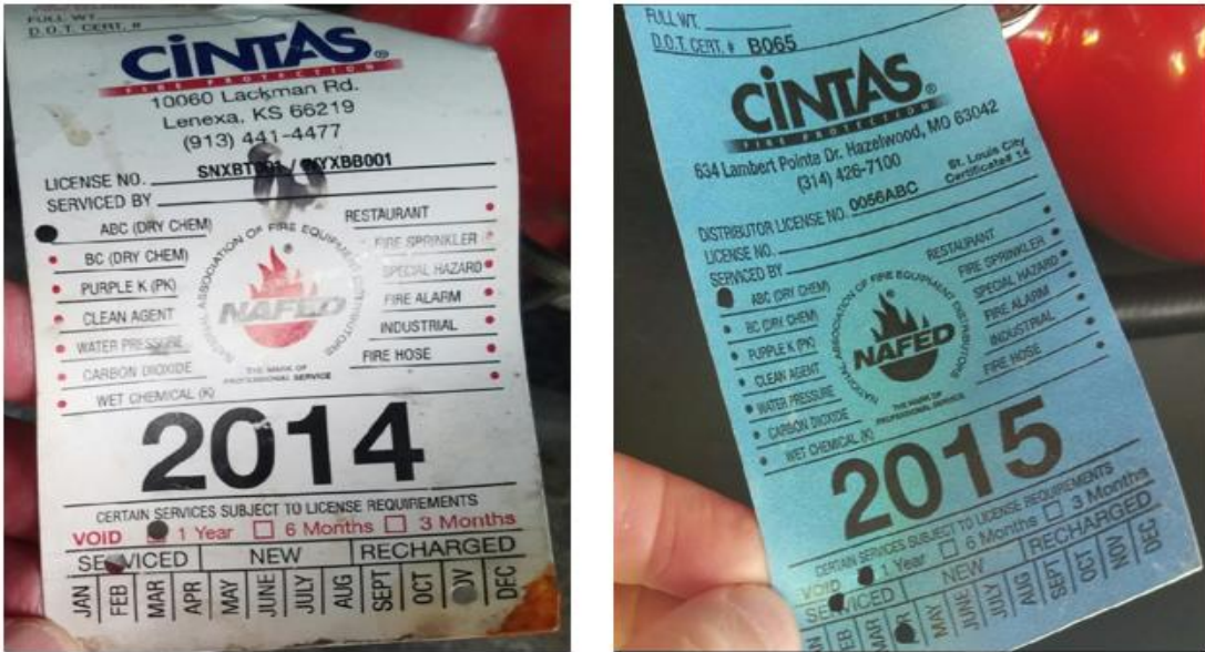
Source: CGCS Team Site Visit
