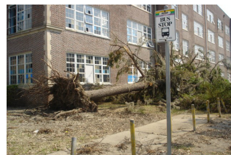
Hurricane Katrina uprooted trees and blew out windows at New Orleans' Fortier High School.
